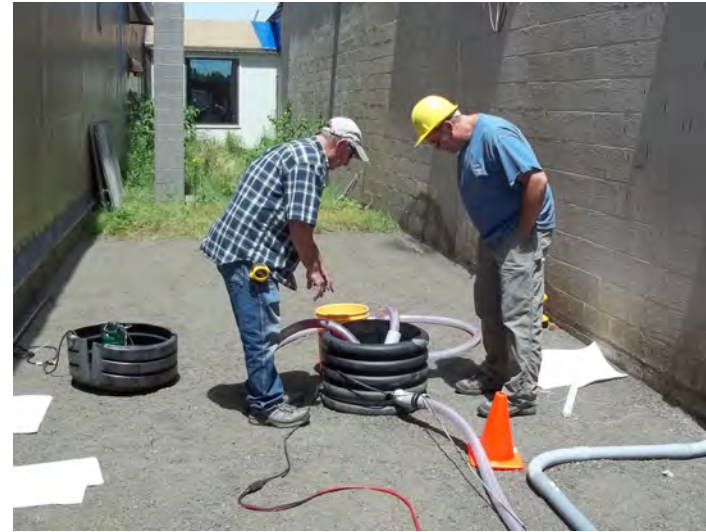
*Rubb Chemical Spill Remediation
